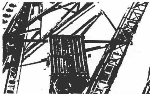
FIGURE 5. PORTION OF FRAMEWORK OF SERVICE TOWER.
