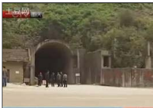
One of the entrances to Project 816
