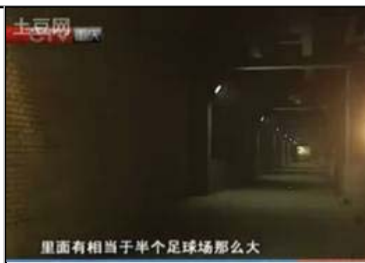
Shot of tunnels inside the underground nuclear facility
