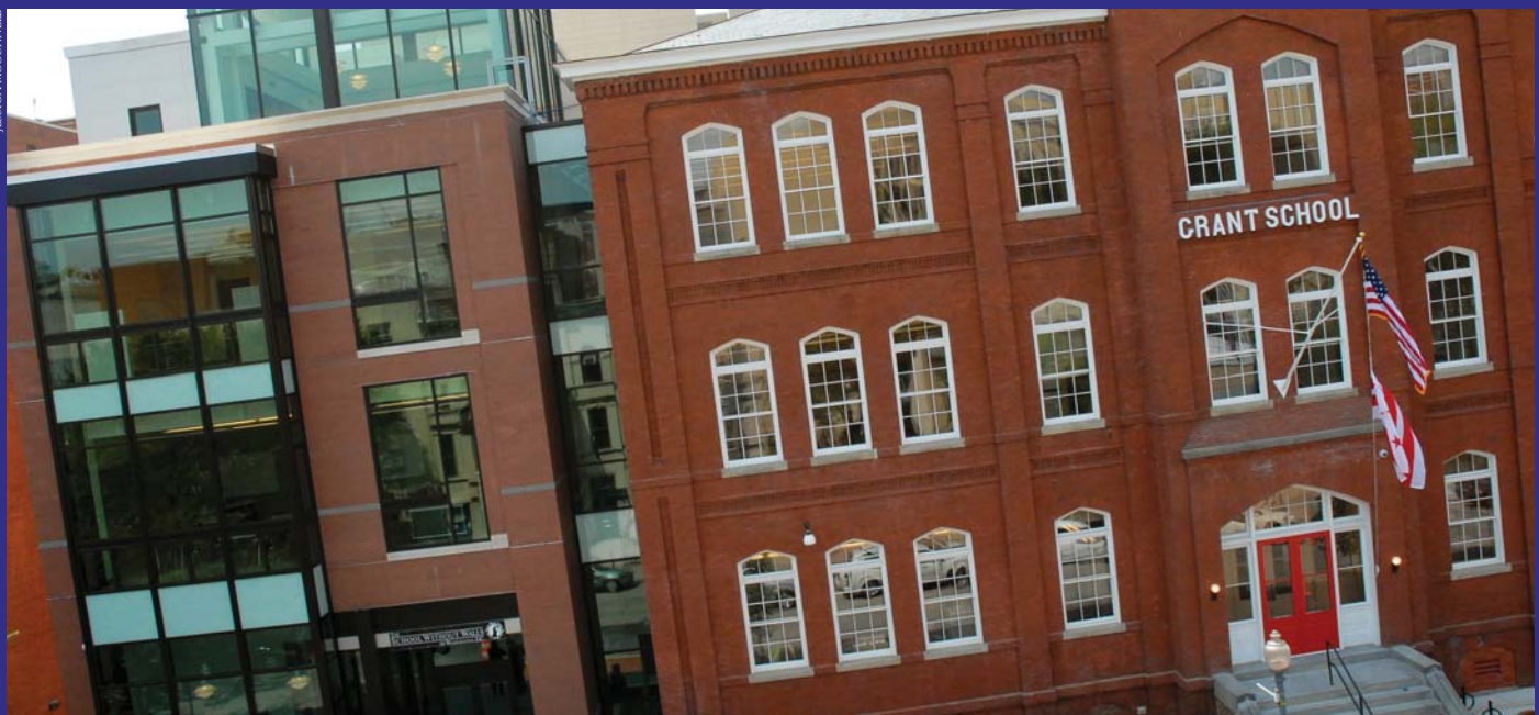
The two-year, $33-million renovation to School Without Walls includes a new 68,000-square-foot, glass-enclosed building that houses up to 100 more students than before. In a development partnership, GW supplied $12 million toward the renovation.
